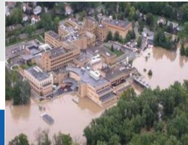
Flooding of Lourdes Hospital, Binghamton NY, 2006
