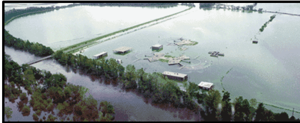
Flooded wastewater treatment plant in Goldsboro, NC (1999)
