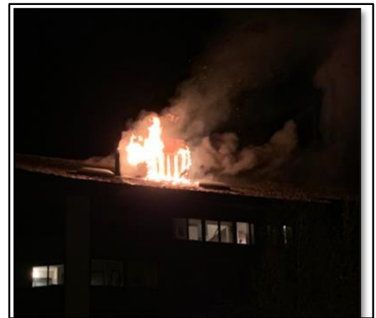
Chimney chase fire on the roof of a five-story commercial and residential complex.
